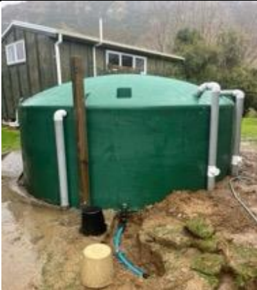
Frances Marshall (TPK – Housing Repairs Water Tank Instalment)
